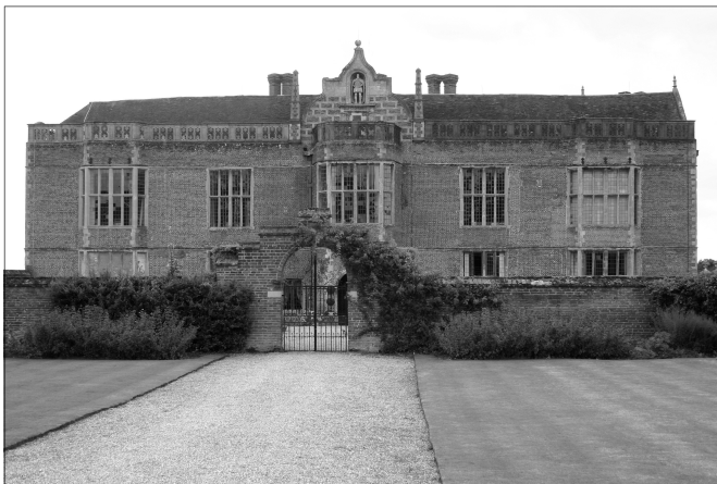
Fig. 1. Bramshill House: the north east side with the figure of Sir Edward Zouche high in the niche.
