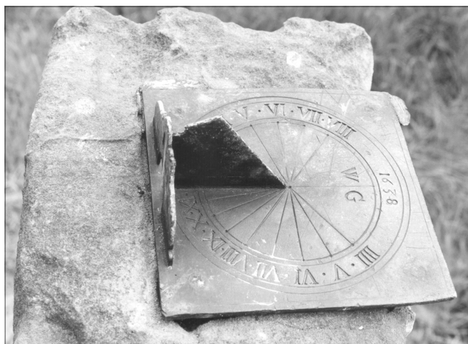
Fig. 2. The dial at Preston Gubbals in 2002. The precarious fastening is clear.
